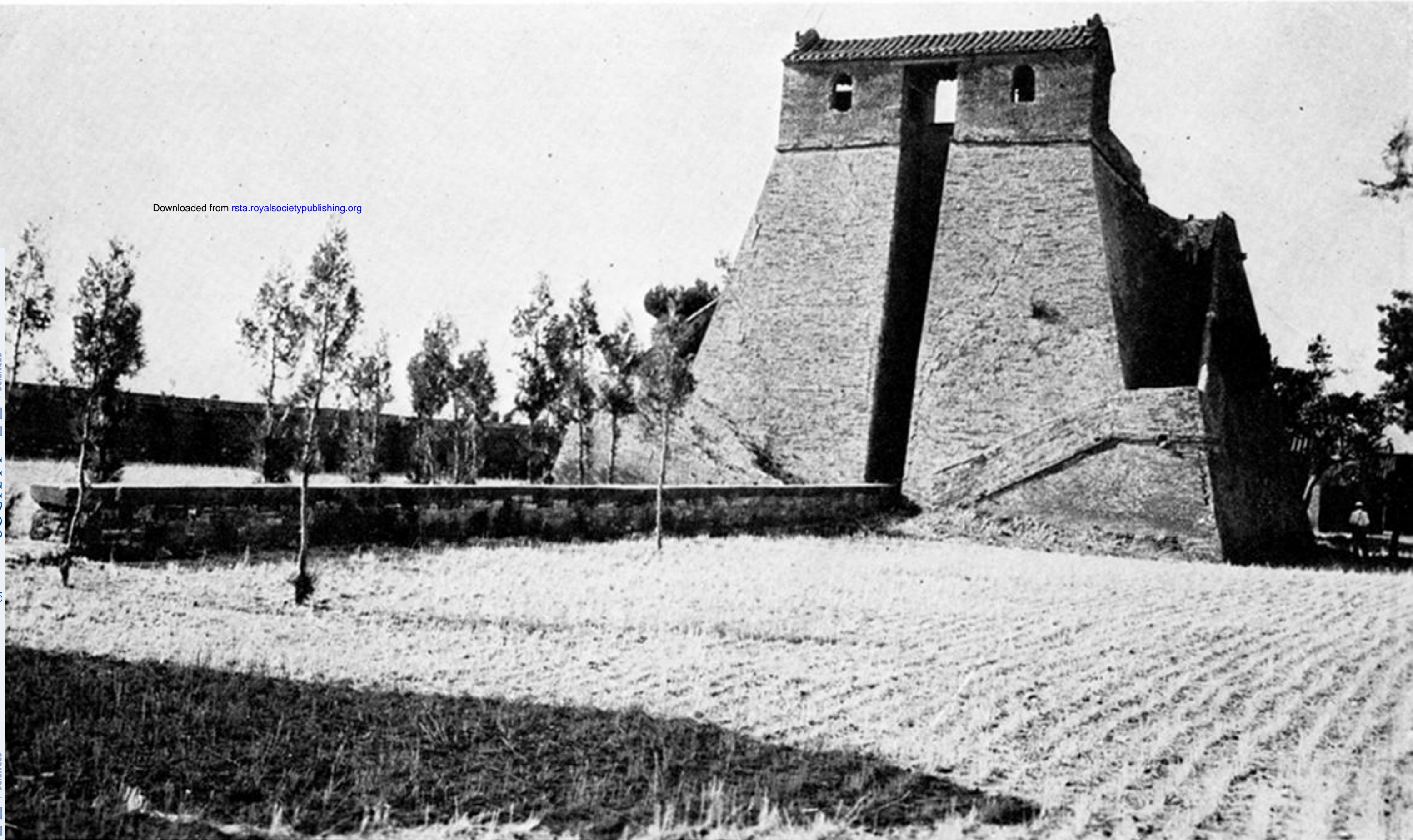
FIGURE 9. The Tower of Chou Kung for the measurement of the Sun's solstitial shadow lengths at Kao-chhêng (formerly Yang-chhêng), some 80 km southeast of Loyang, and for many centuries the site of China's central astronomical observatory. The present structure is a Ming renovation of the instrument built by Kuo Shou-Ching about +1276. The 12 m gnomon stood up in the slot, and its shadow was measured along the stone scale projecting on the left, with special arrangements to secure a sharp edge reading. One of the rooms on the platform housed a clepsydra (perhaps a hydro-mechanical clock), and the other probably an observational armillary sphere.
